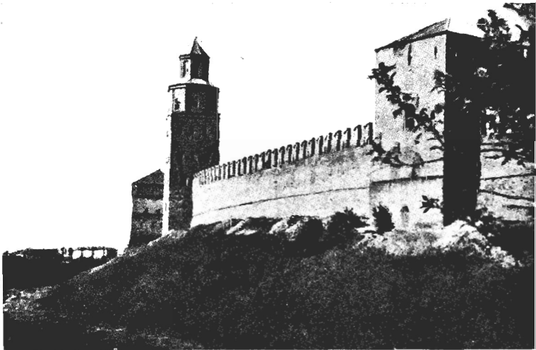
FIG. 13.—Novgorod Kremlin. Walls and towers built anew at the close of the 15th century. Superstructure added to the high Kokui tower in the 17th century. (Phot. APN.)
